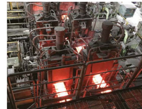
One heat process shortens the casting process
