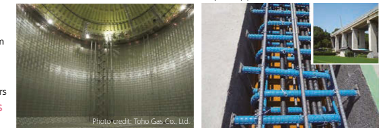
Internal stairs inside LNG tank (low ductility in low temperatures)
