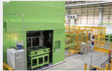
Electronic component line No. 3 completed in October 2022 in response to high demand accompanying an increase in electrified vehicles
